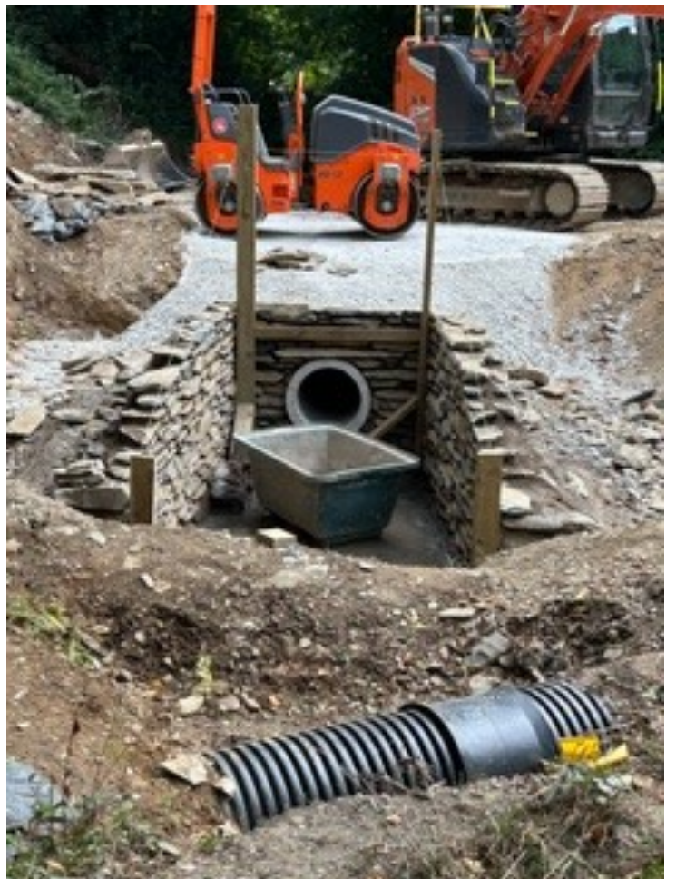
The stream diverted via the large black tube
